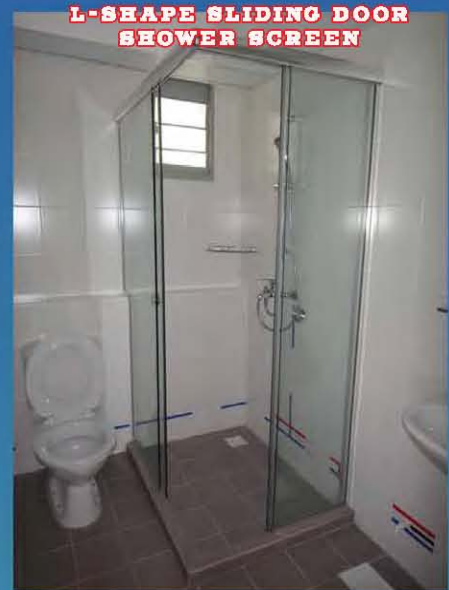
GLASS TO GLASS WITH TOP REINFORCEMENT STAINLESS STEEL BAR
