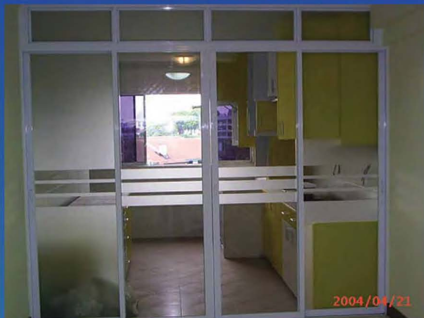
SLIDING DOOR WITH TOP FIXED PANEL
